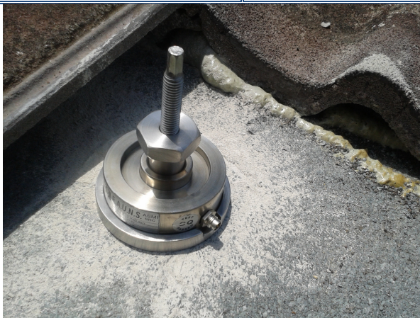
1. Test of Extraction
