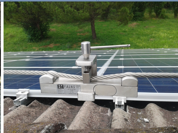
2. Rope tensioning
